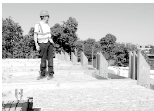
Working on the First Floor
